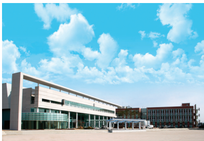
Technical Training Center in the GIC
