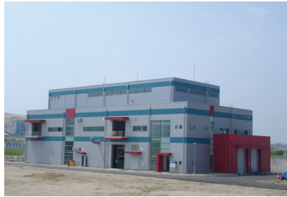
GIC waste incineration facility
