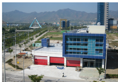
GIC fire station
